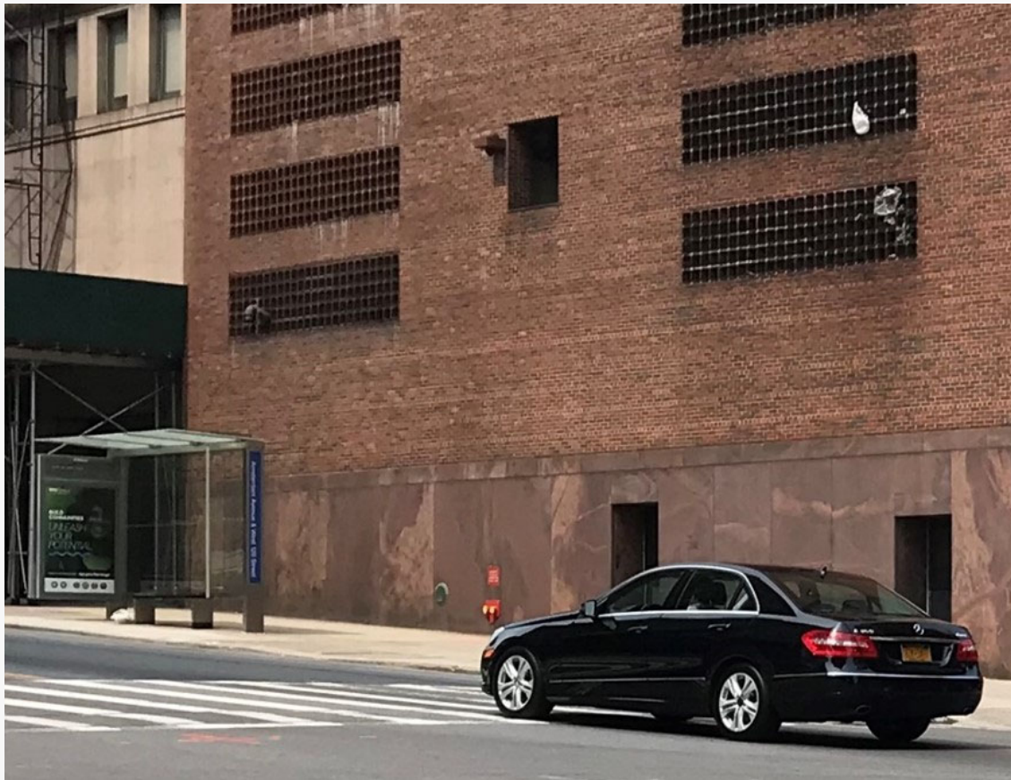
COSMOS node with camera as viewed from across Amsterdam Avenue
